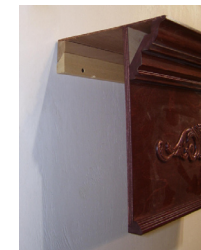
3. Hang cornice on the cleat and center over the window.
