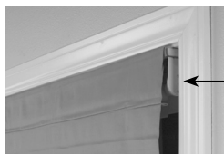
Partially recessed headrail in window casing/molding
